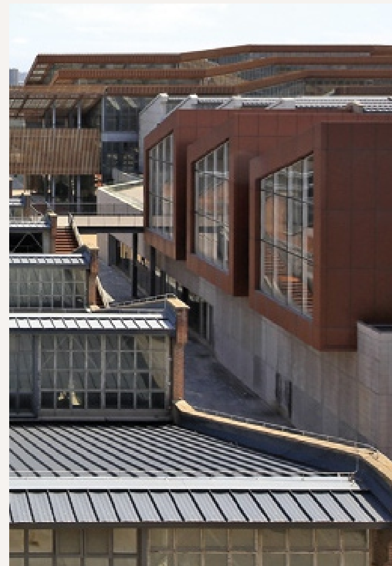
Renovation of Xi'an Dahua Textile Mill / D.R.C
