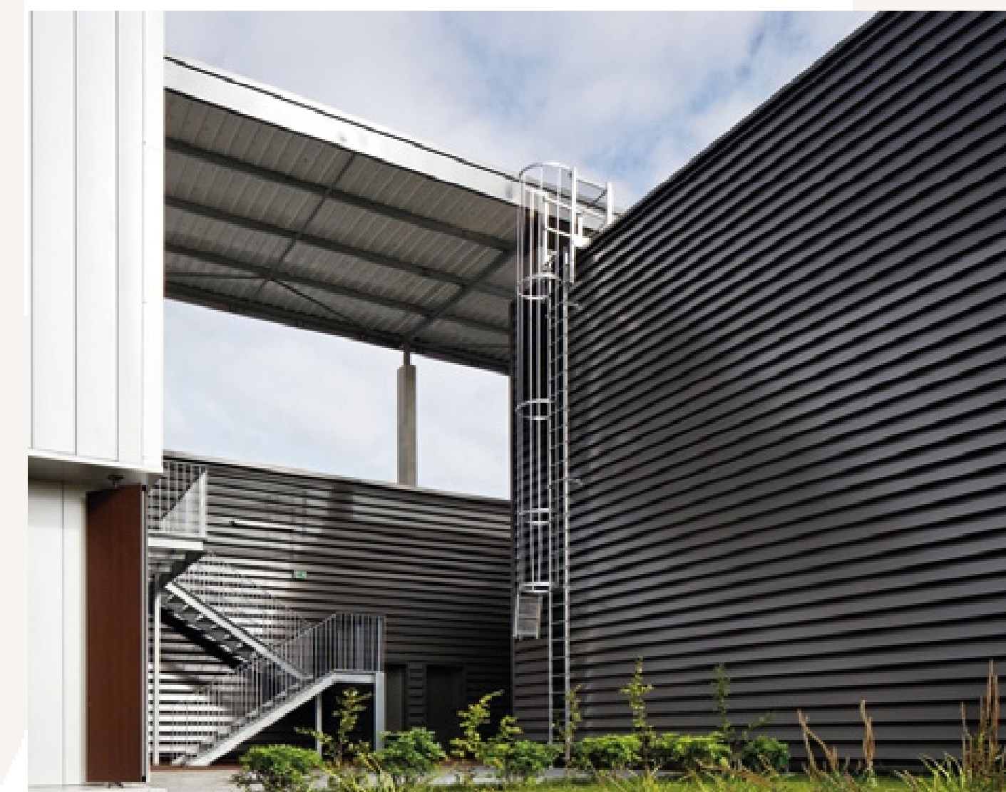
Municipal Technical Center / STUDIOS Architecture
